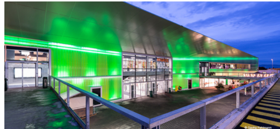
Centre commercial Migros Romanel
